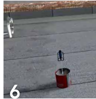
6 Mix the membrane with STARFLEX MEMBRANE for 3 minutes
