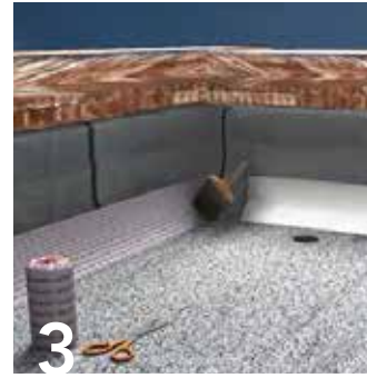
3 Treat all joints and cuffs with STARTEX NW DETAILS fabric
