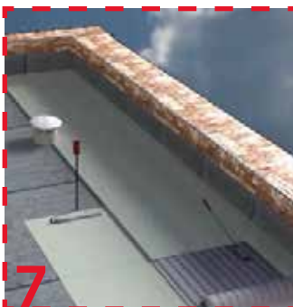
7 In case of reinforcement, apply two layers of one-component STARFLEX membrane with the reinforcement in between STARTEX optional
