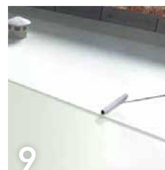
9 Optionally apply a non-yellowing finishing layer STARFLEX MONO TOP or POLISTAR E/P
